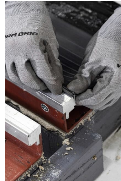
Ref 23. Insert the tie-in wing dart of the WJS gland into the receiver channel, taking care not to stretch the material while doing so. A rubber mallet can be used to assist with getting the gland fully inserted into the channel.
