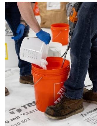
Ref 8. Add Tremco PUMA Polyethylene Fiber to flashing-aggregate mixture while the mixer is running.
