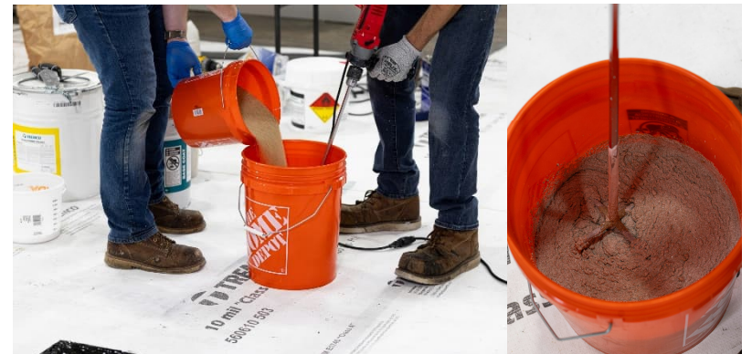
Ref 7. Add Aggregate to pre-mixed Tremco PUMA Flashing and mix for 1 to 2 minutes with egg-beater style paddle.
