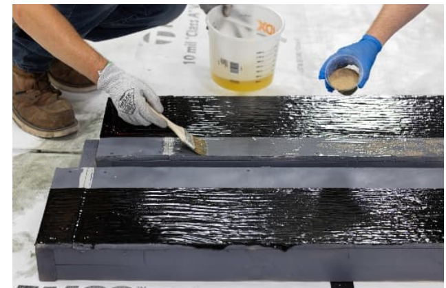
Ref 5. Apply Tremco PUMA Primer and lightly broadcast silica sand into the primer.
