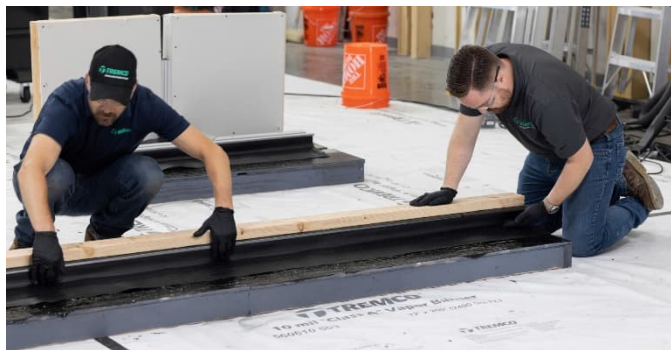
Ref 46. Carefully place rubber tie-in wings into the wet (uncured) initial lift of fluid-applied waterproofing.
