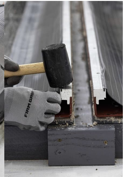
Ref 23. Insert the tie-in wing dart of the WJS gland into the receiver channel, taking care not to stretch the material while doing so. A rubber mallet can be used to assist with getting the gland fully inserted into the channel.
