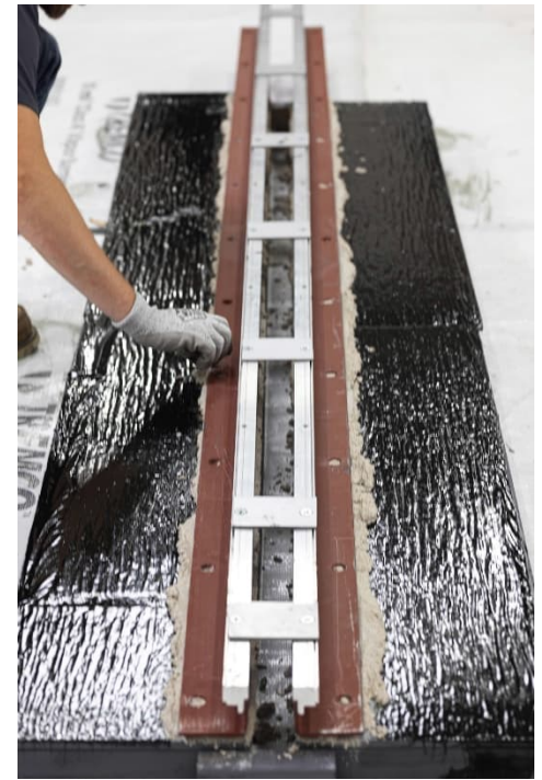
Ref 16. Remove excess setting bed material that has migrated out from under the areas required for bracket support before it cures.
