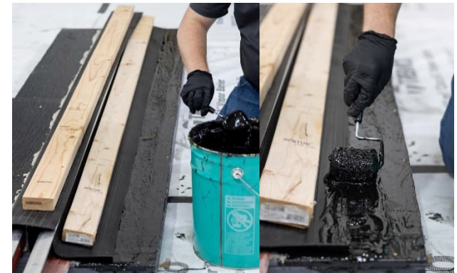
Ref 47. Install the second lift of fluid applied waterproofing material at thickness of 45 wet mils. Ensuring coverage extends out 1/4" to 1/2" margin to completely encapsulate the rubber tie-in wing between the two layers of waterproofing.
