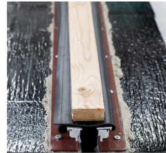
Ref 41. Secure rubber wings up and off the bracket, setting bed, and tie-in areas when applying waterproofing.
