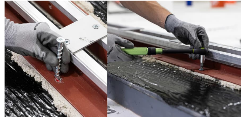
Ref 21. Install anchor bolt into each bolt hole with epoxy capsule inserted.
