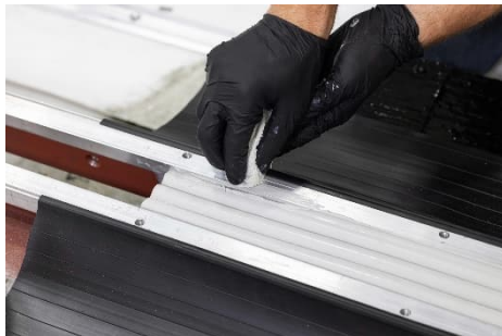
Ref 39. Clean off any foam detail sealant that may have migrated onto the brackets.
