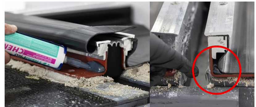
Ref 43. Gun a liberal amount of TREMPRO Chem-X Pro into the void at the bracket upturn.
