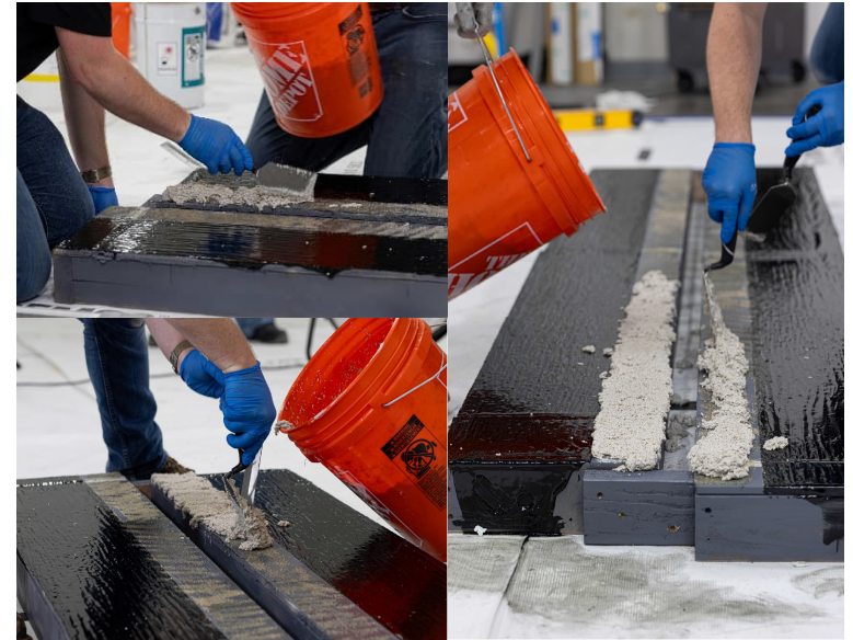
Ref 10. Use a mortar or mason's trowel to apply the setting bed to the bare, properly prepared and primed concrete.
