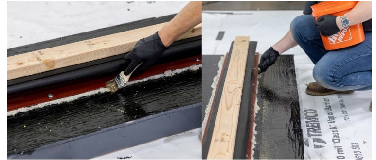
Ref 44. Apply a coating of TREMprime VB+ epoxy primer to the tie-in area beneath the rubber wing and lightly broadcast with industrial grade silica sand.
