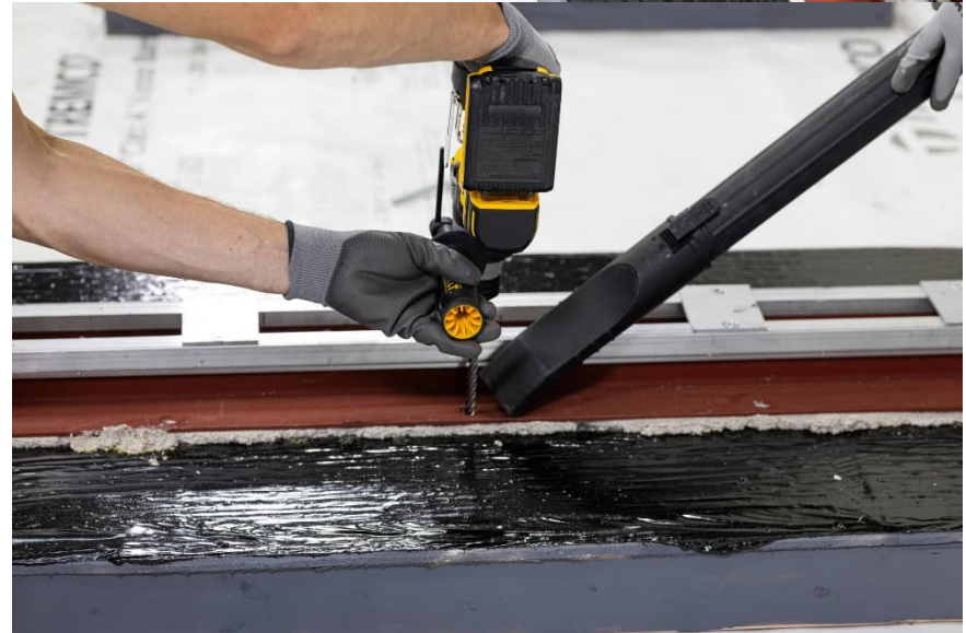
Ref 19. Use Shop Vacuum to remove dust from inside and around anchor holes when drilling.
