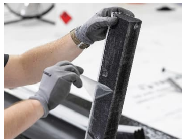
Ref 31. Remove the release liners from the stick of foam.
