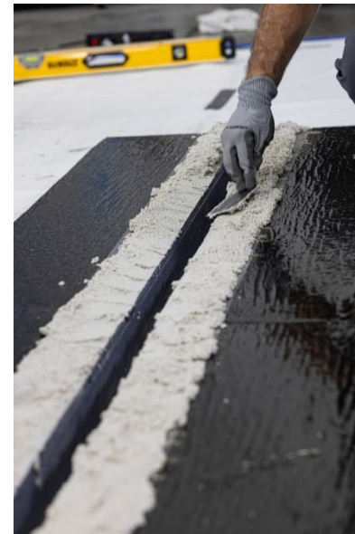
Ref 11. Ensure that the finish of the setting bed is uniform.
