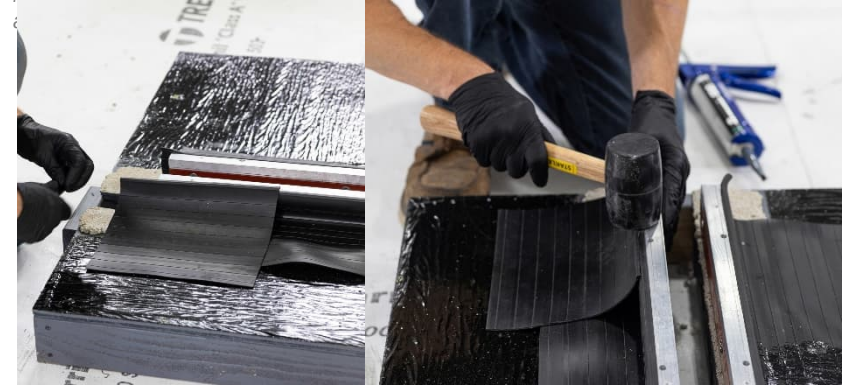
Ref 25. Align and install the sections of Willseal WJS gland that will overlap, making sure the rubber darts are even and there is 2" of overlap between the sections.
