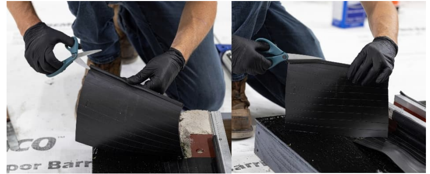
Ref 24. Trim 2" of dart off one connecting end of the Willseal WJS gland, ensuring the butt ends
