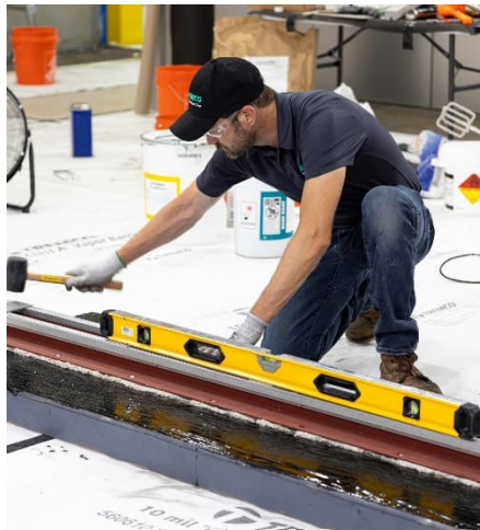
Ref 13. Using a rubber mallet, tap the rails into the setting bed until the desired height has been achieved.
