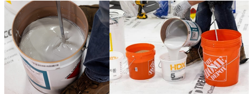
Ref 6. Pre-measure all PUMA Setting Bed components and pre-mix Tremco PUMA Flashing before adding aggregate.
