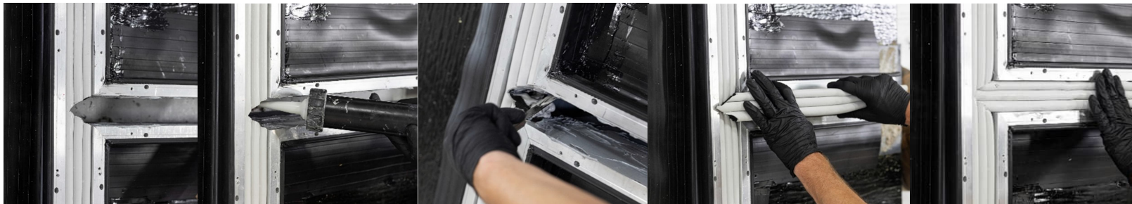
Ref 35. Create a T-intersection by cutting a notch out of the straight run of foam and cutting the adjoining stick into a point, matching the angle to the notch. Apply the supplied foam splice adhesive to both sides, tool ensuring both the notch and point are fully buttered. Then press the pieces of foam together while maintaining compression along the joint.
