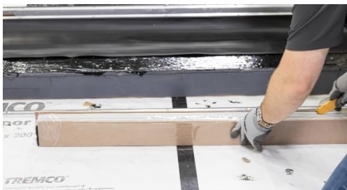
Ref 30. Carefully cut/slit the shrink packaging along the edge of the masonite strapping.
