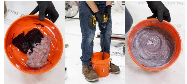
Ref 28. Mix the supplied epoxy at a 1:1 mixture of part A and part B. The epoxy can be mixed by hand or using a high-speed mixer. Mix both parts together until the mixture is a uniform gray color.
