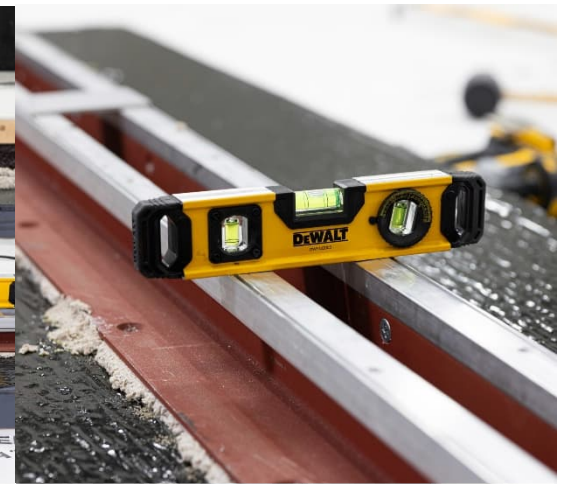
Ref 14. Using 4ft, 2ft, and torpedo levels, confirm that the brackets are level across the width of the joint, from bracket to bracket, and through the length of the joint along each bracket.
