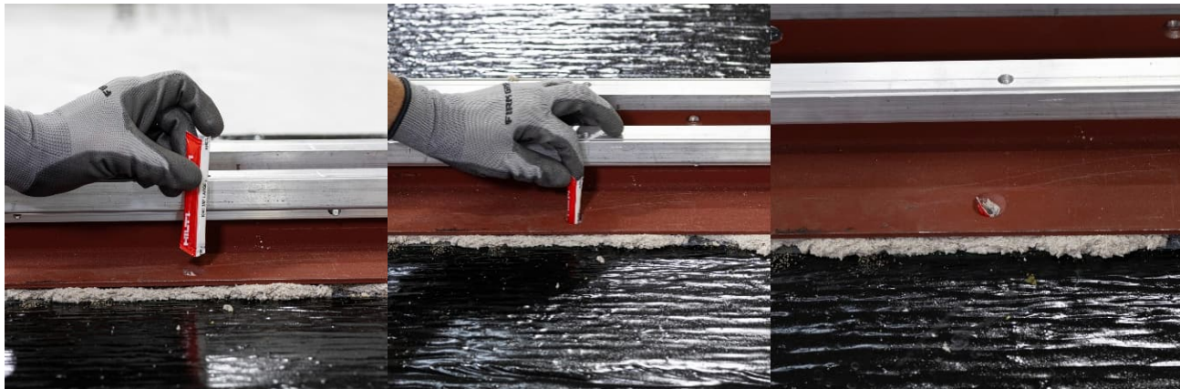
Ref 20. Insert and fully seat epoxy capsule into each anchor bolt hole. The top of the epoxy capsule should be flush with the top of the hole.
