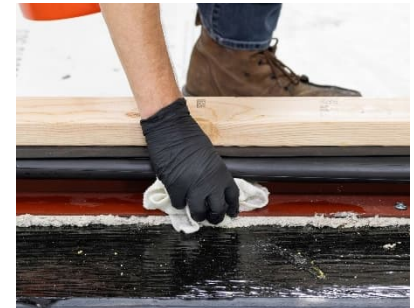
Ref 42. Clean all exposed surfaces of Willseal MSS setting bed with PUMA Cleaner.
