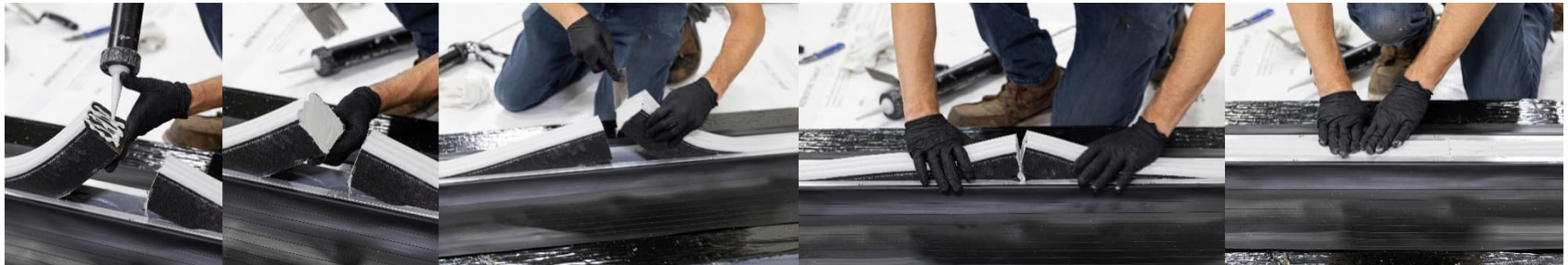
Ref 34. Apply the supplied foam splice adhesive to both ends of the connecting sticks, tool ensuring both ends are fully buttered. Then press the two ends into the joint together.
