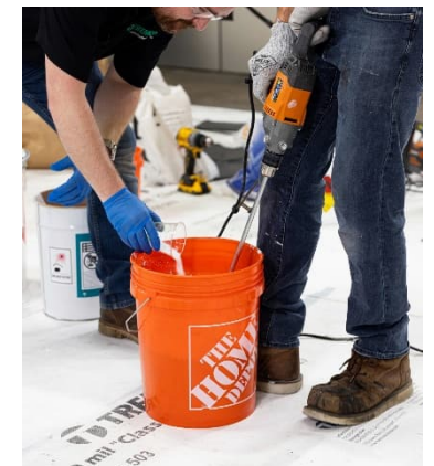
Ref 9. Split dose of Initiator+ in half and mix one half at a time into mixture until full dose is added.
