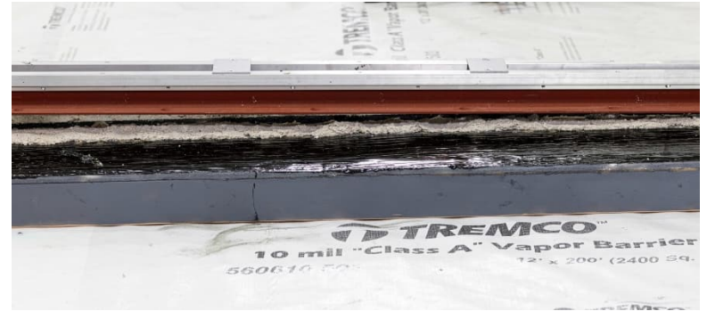
Ref 12. Place the first length of metal brackets into the wet setting bed material.
