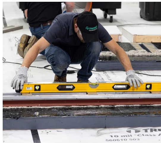
Ref 14. Using 4ft, 2ft, and torpedo levels, confirm that the brackets are level across the width of the joint, from bracket to bracket, and through the length of the joint along each bracket.
