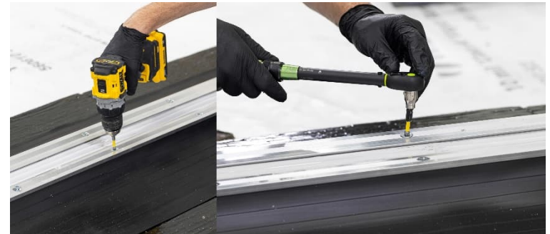
Ref 40. Reinstall the flat-head top cap strip screws with a Phillips head bit and torque to 60 in-lbs (5.2 ft-lbs; 7 Nm).
