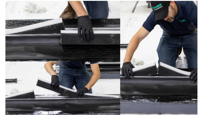
Ref 33. Install each subsequent stick of foam in compression against the stick previously installed, by installing the two sticks with an overlap in the material.
