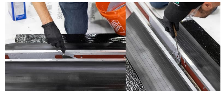
Ref 29. Apply fully mixed epoxy to both bracket sidewalls at a 1/16" to 1/8" thickness for the full depth of the foam plus 1/2".
