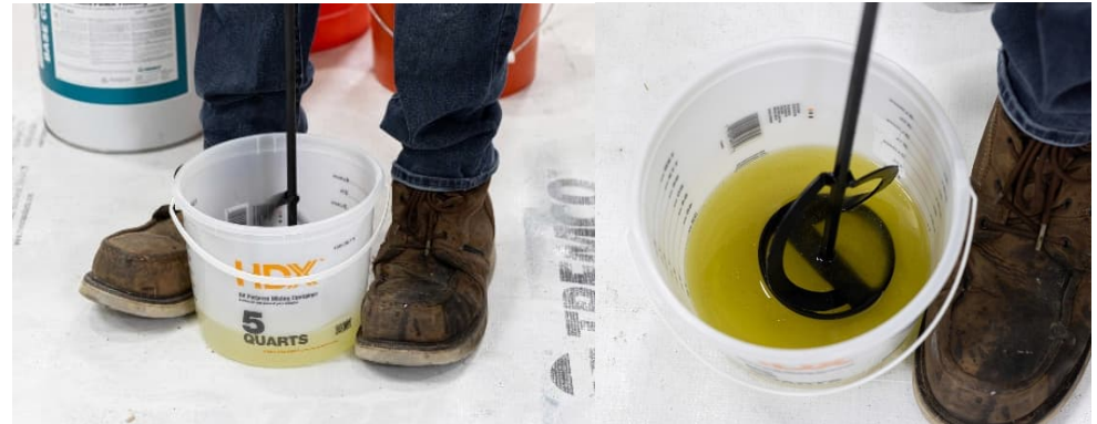
Ref 4. Mix Tremco PUMA Primer and Tremco PUMA Initiator+ together for 2 to 3 minutes.
