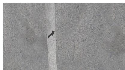
Ref 2 – Ensure depth for ¼ in. foam recess minimum.
