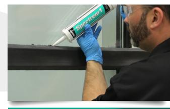
Silicone Dense Rubber Extrusions—custom designed, patented solution for restoring leaking skylights, sloped glazing, pressure bar and zipper/ lockstrip systems
