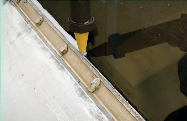
Application of Spectrem 2 sealant on the skylight above the Mayfield Toyota Ice Palace
