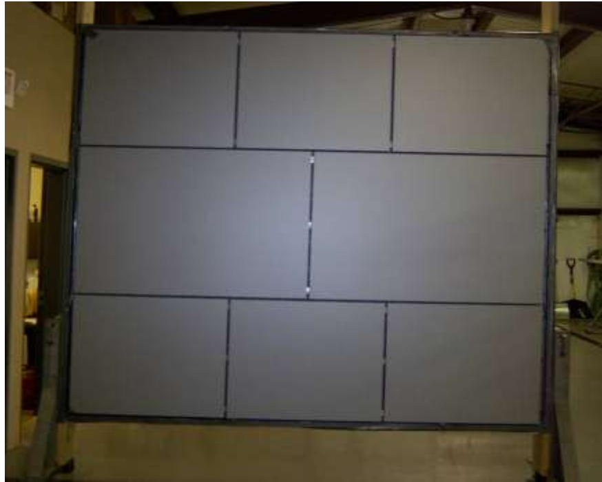
Photo No. 3 ExoAir 230 Control Wall with ACM 4100 Panels
