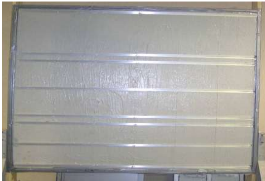
Photo No. 2 ExoAir 230 Control Wall with aluminum angles
