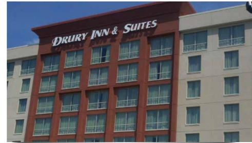
*After pressure washing the entire building below, HDP Coating was applied to only the left portion of the building. Five years later, it is still clean while the right side — without HDP Coating — shows the wear from normal environmental conditions.*
