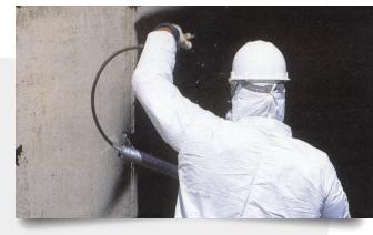
The WATCHDOG Waterproofing membrane is spray-applied to seamlessly bridge shrinkage cracks and seal out water penetration. Its material was specifically designed for spray application on below grade exterior foundation walls. The membrane remains elastic at low temperatures for dependable year-round protection.
