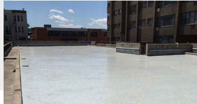
Completed System Prior to Asphalt Topping
