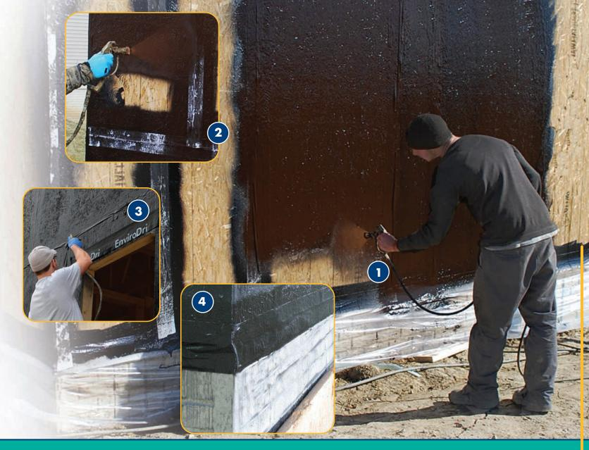
The Enviro-Dri Weather-Resistant Barrier System is comprised of four integrated components that work as a unit to seal and protect the building envelope:
