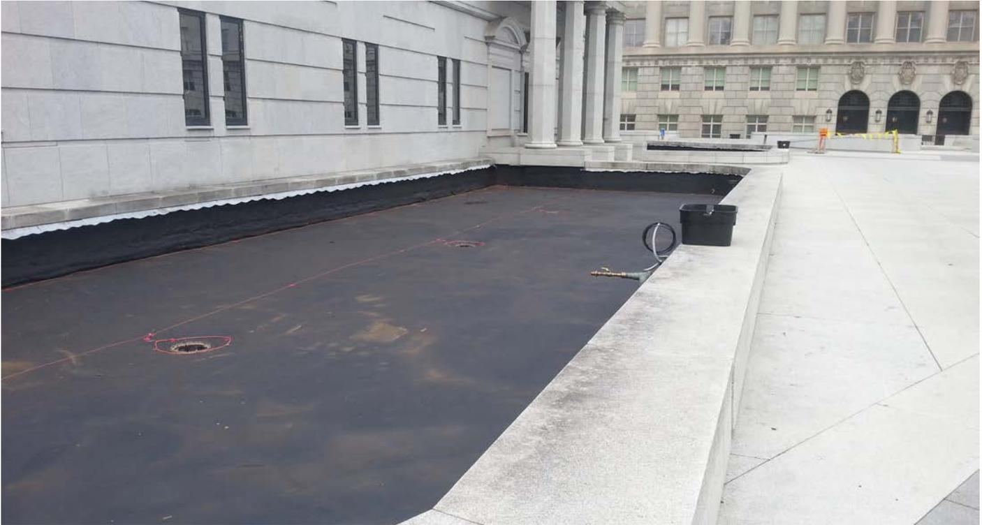
About half of the project included planters and 40,000 square feet of vertical surfaces so the TREMproof 250GC with its trowel-grade version helped to ensure no areas were left untreated or exposed to moisture infiltration. TREMDrain GS drainage mat was used over the membrane to enhance the performance of the waterproofing system by functioning as a water retention layer while designed to also prevent root growth.
