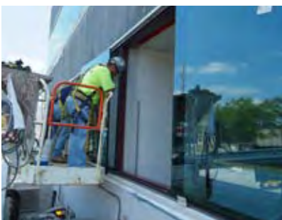
Tremco setting blocks were positioned at the sill of the window to support the weight of the energy-efficient insulating glass unit and provide the correct glass "bite" or depth within the assembly for a comprehensive, compatible system designed for long-term performance.
