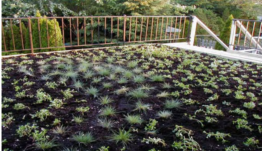
Figure 1: A Typical Green Roof. Green roofs have many ecological benefits including heat island reduction, storm water management and the plants convert carbon dioxide into oxygen.
