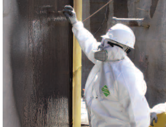
Today, the solids formulation in spray-applied waterproofing membranes maintains consistency of the sprayed product, and approved contractors will routinely gauge wet mil thickness to ensure architects' specifications are met.
