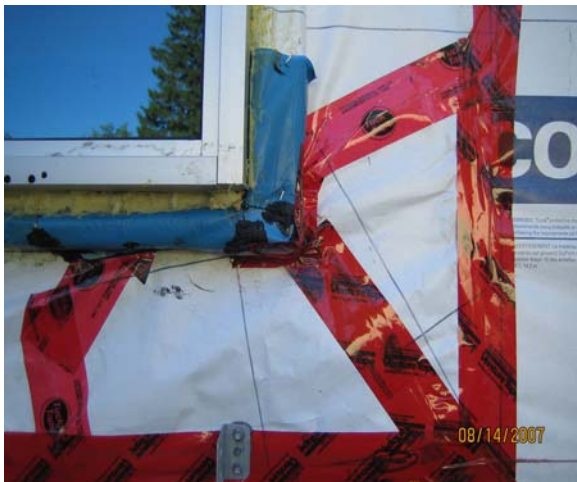
Figure 3. Commonly found deficiencies at window-wall interface. Top photo shows reverse-shingling of building paper and membrane wrap. Bottom photo shows PVC flange not secured flush to the wall and membrane wrap poorly detailed and not fully adhered to the wall air/vapor barrier membrane.
